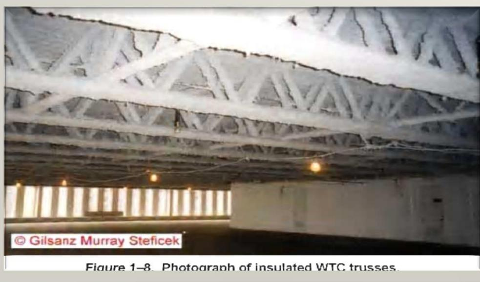
Figure 1-8. Photograph of insulated WTC trusses.
